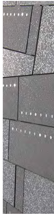
GREAT PAVING THROUGHOUT
